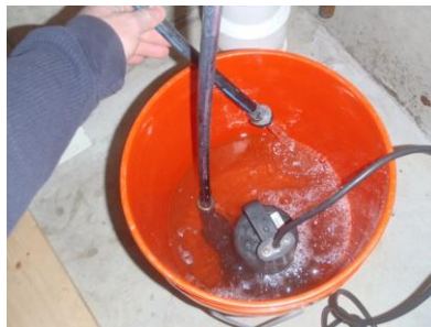
Flushing with vinegar
